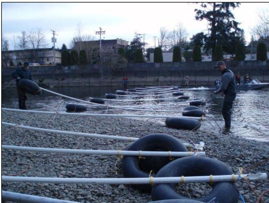
**Photo 1.** Assembling and installing the 3-cable array, April 2008. Photo looking from east to west shore (river left to river right) at low tide.
